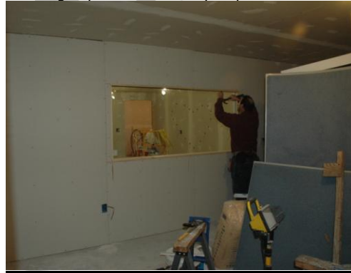
Viewing window into the nursery is installed
