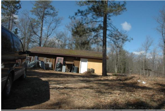
Garage with building site right and behind
