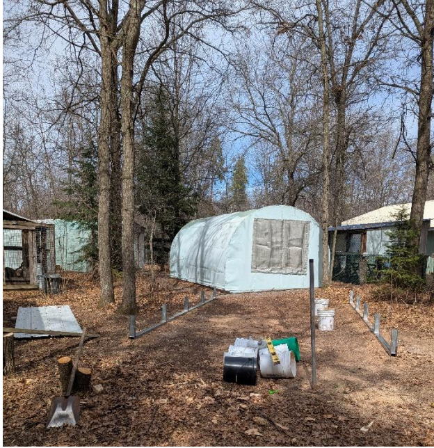
Base and uprights are laid out.
