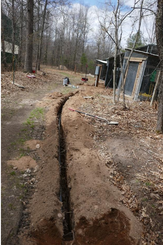
New electric lines being installed
