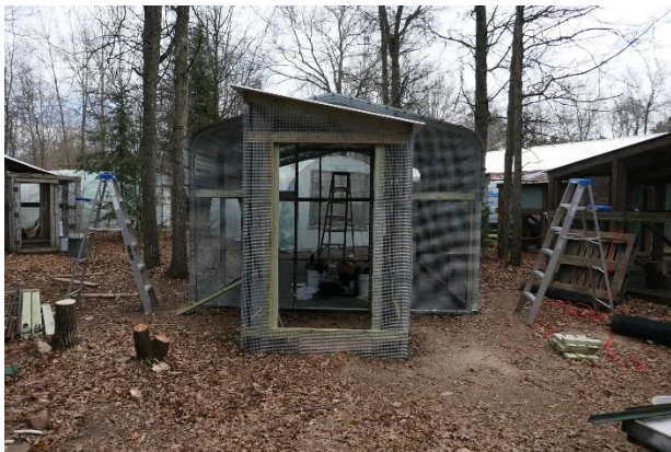
Almost complete, needs doors & substrate.
