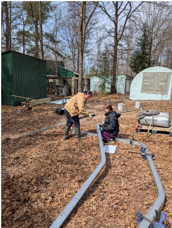
Intern Karina & Heather assemble trusses.
