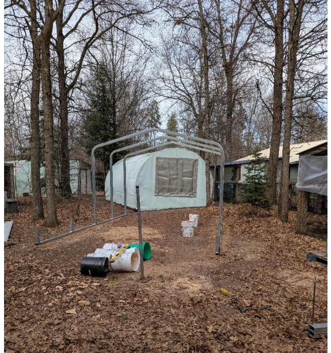
Trusses being erected.
