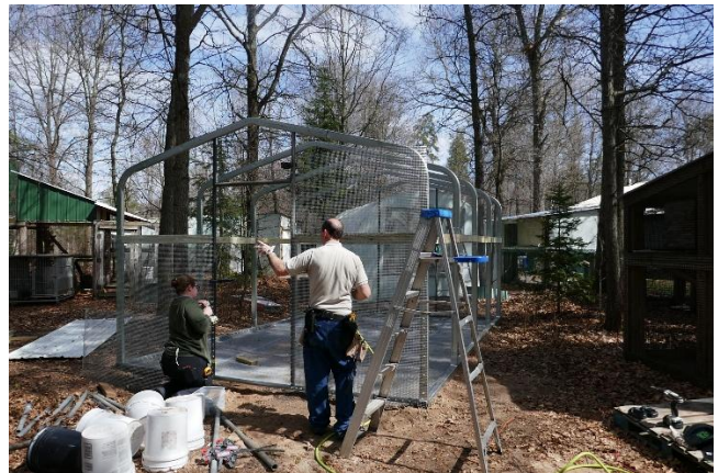
One layer of sidewall being installed.
