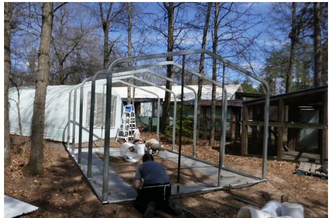
Predator proofing being installed.
