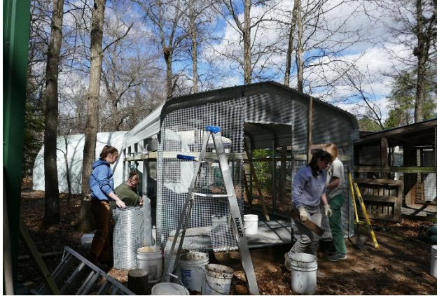
More sidewall being installed.
