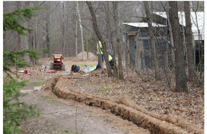
Electricians hard at work.
